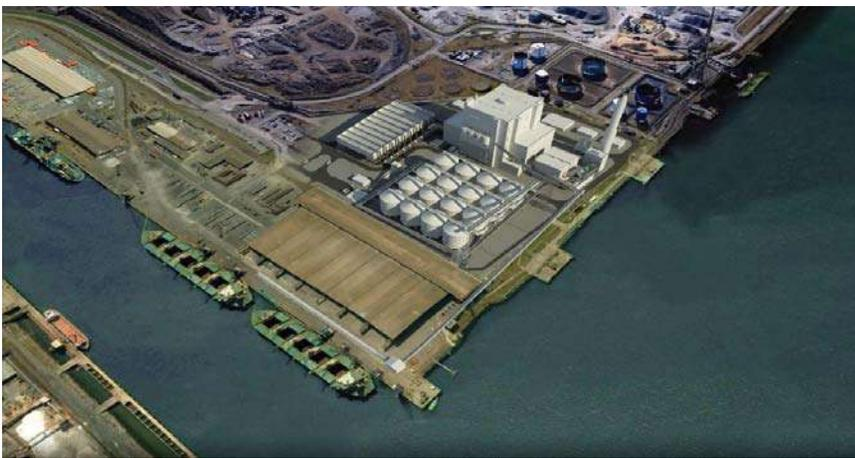
*Note: The Teesside plant is built around a Sumitomo SHI FW CFB boiler and a single steam turbine. It also comprises a fuel storage area and conveyor system, a wood chip drier and an air-cooled condenser.*
