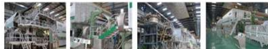
PM 7 After Project Completion
