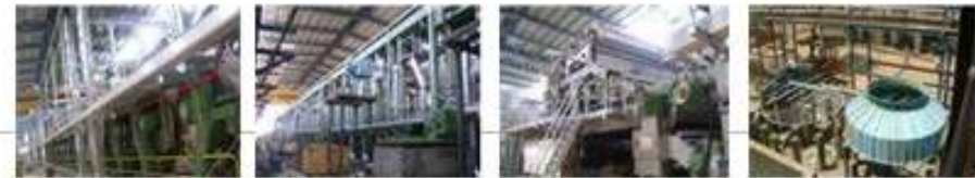
Mechanical Erection Work at Site
