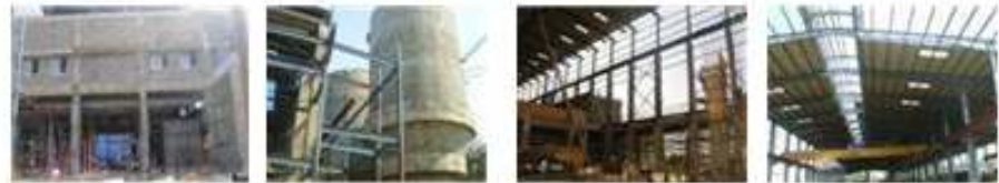
Various Stages of Civil Work at Site
