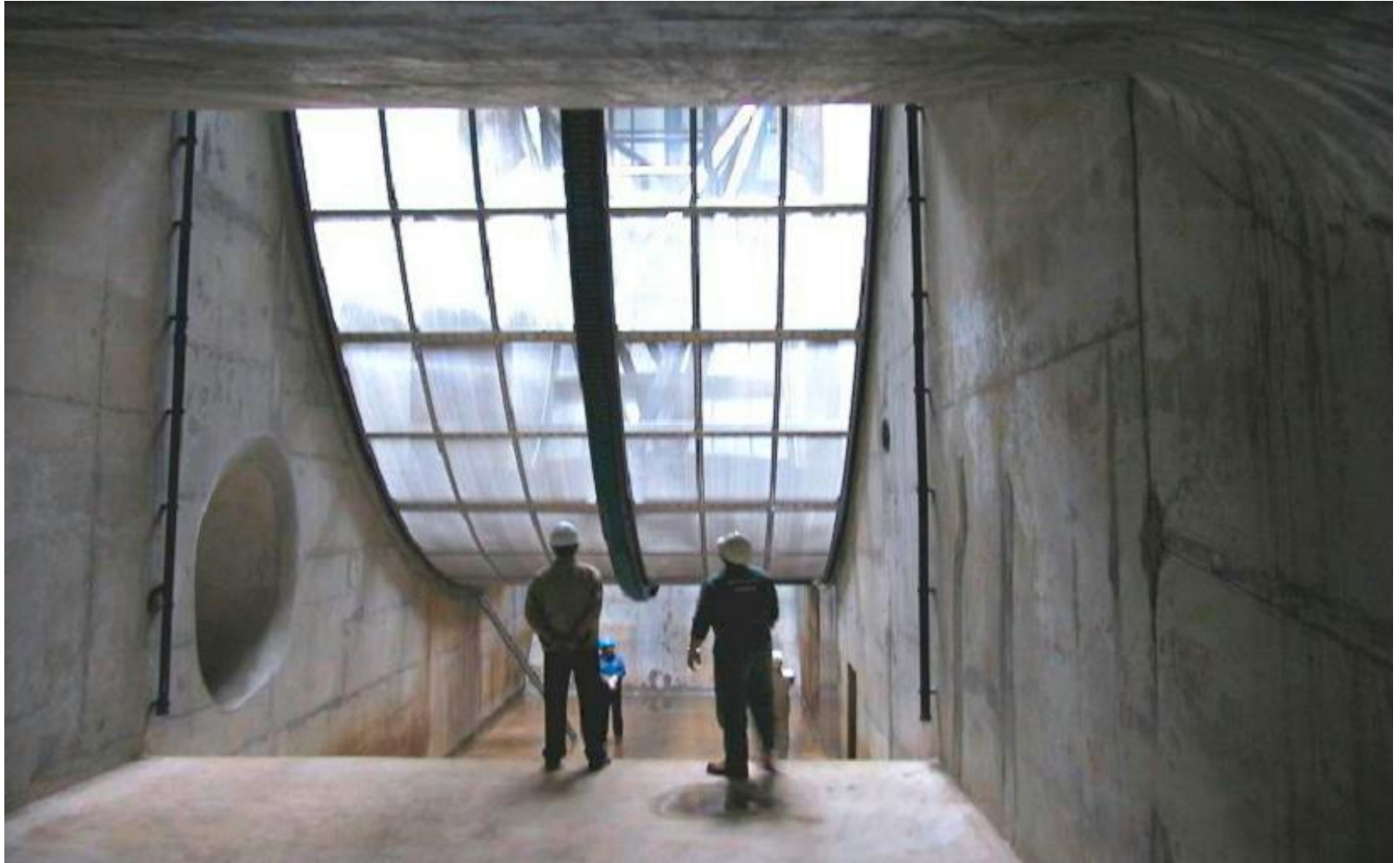
Looking out from the CW intake underneath Drum screen - Lingo Ao NPS, China
