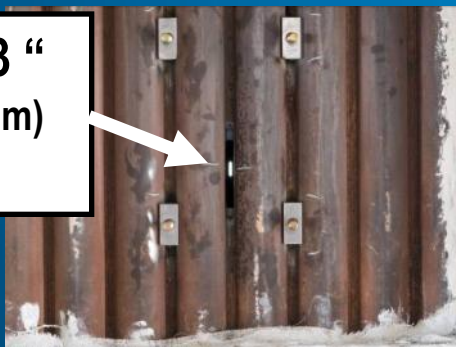
Slotted Opening in Membrane
