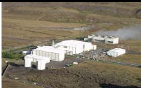
Geothermal Power Plant
