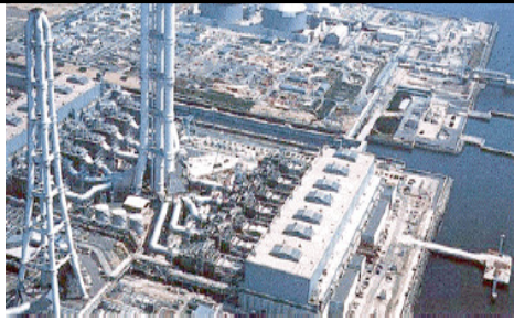
Combined Cycle Power Plant
