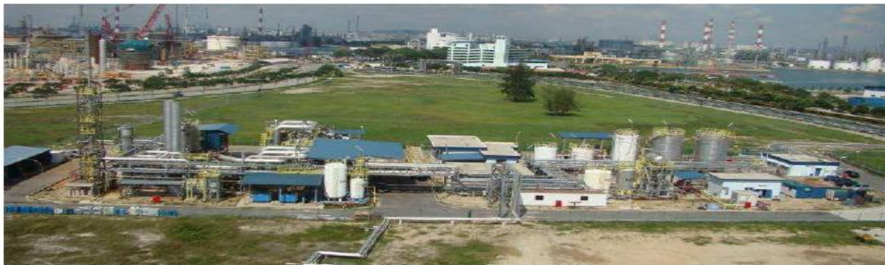
Plant 15 MWth - Jurong, Singapore
