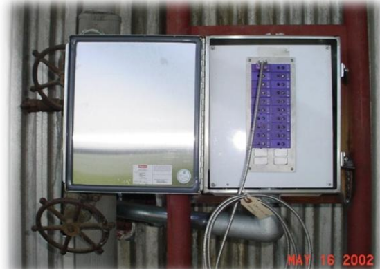
Primary Super-Heat (PSH) Element Tube Metal Thermocouple Installation
