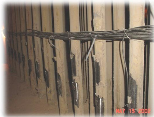
Primary Super-Heat (PSH) Element Tube Metal Thermocouple Installation
