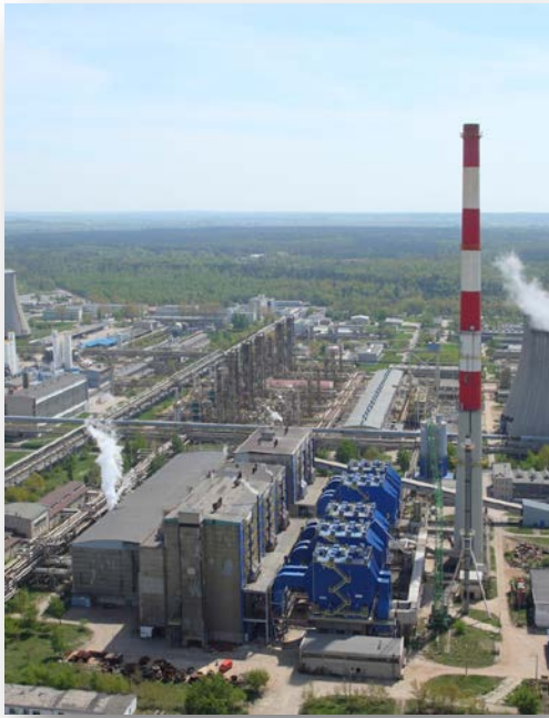
ZAP | Poland (under construction)
