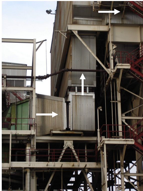
Photograph of duct work between air preheater (APH) exit and ESP inlet
