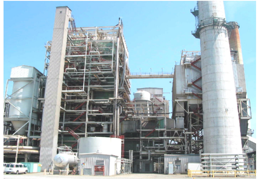
Progress Energy Lee Station, Unit 3
