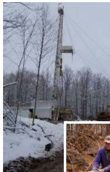
5000 Foot Deep Test Well Drilled in November 2006
