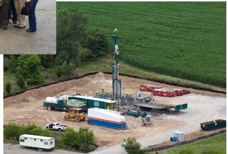
Drilling Operation – Summer 2009
