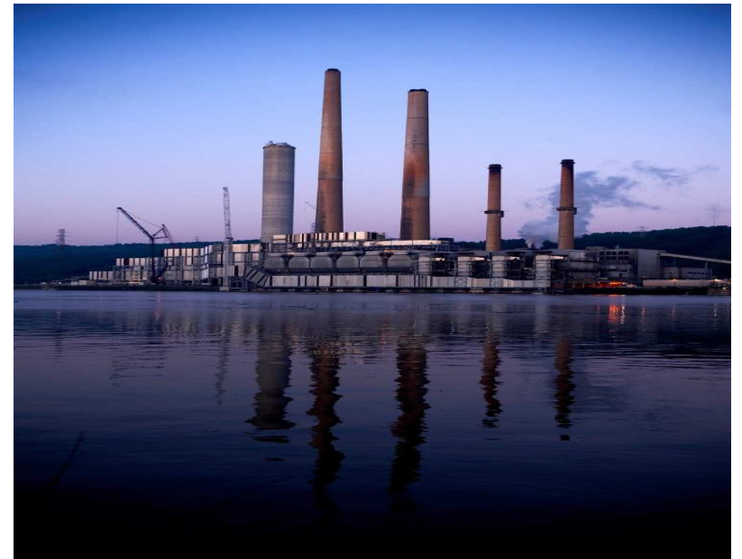
Sammis AQCS Retrofit Project Photo Courtesy Bechtel Power Corp
