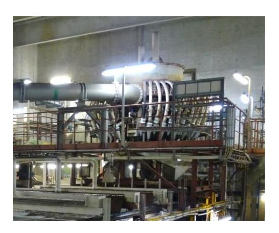
The gypsum handling system consists of a hydro cyclone thickening the gypsum slurry ...
