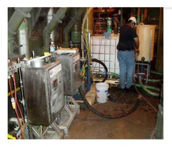
CFD modeling indicates best injection sites (2 nozzles at each of the OFA and Side Door ports). Above shows the pump skids and day tank.
