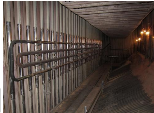
2 nd Steam Loop Installation
