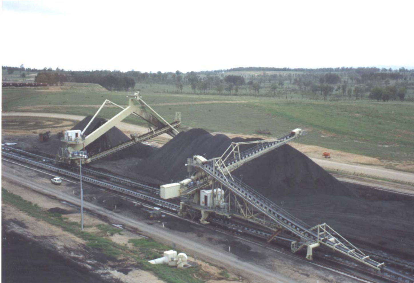
Stacker and Multiple Purpose Reclaimer (front and side reclaiming)
