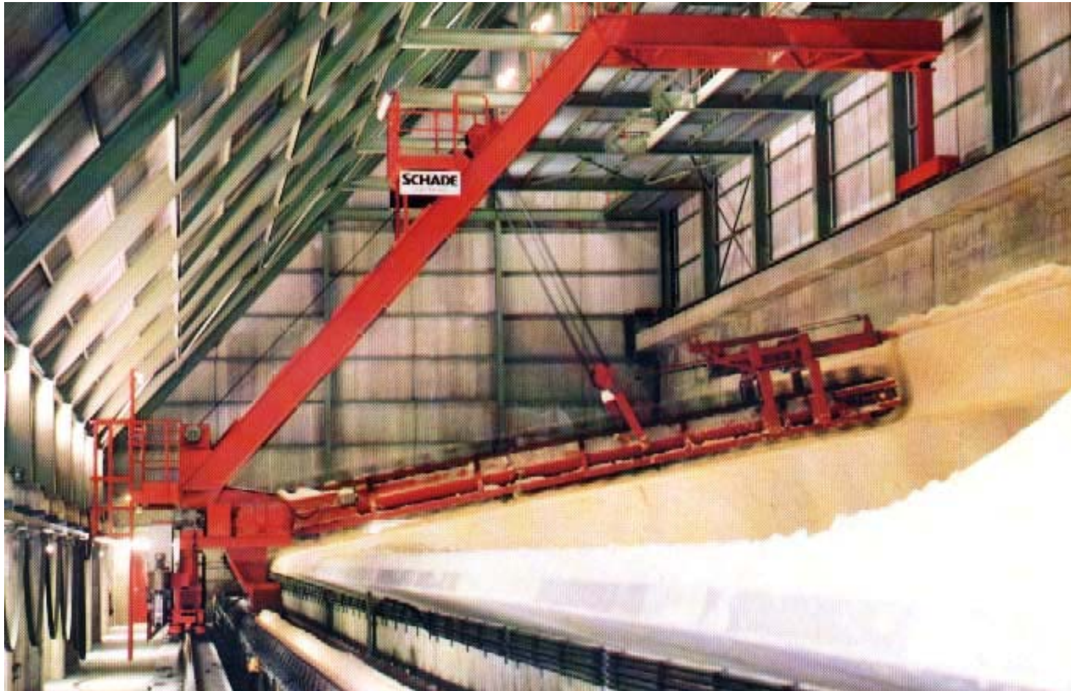
Semi-Portal Reclaimer (discharge via concrete ramp)
