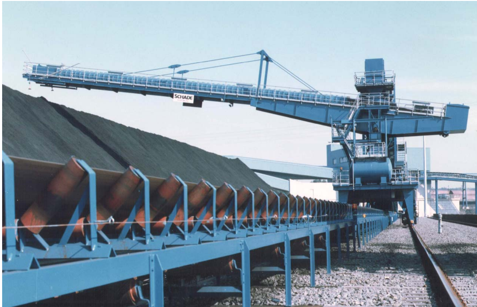
Stacker, slewing and luffing (hydraulic)
