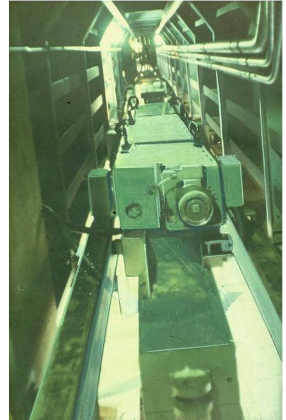
RDM-BL 3000; 11 kW, 200 t/h limestone and marl LEUBE, Austria
