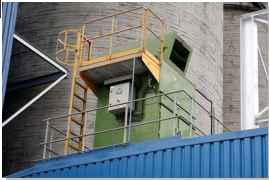
Integral Dust Plant with Filter Bag Housing above the Samson Enclosure
