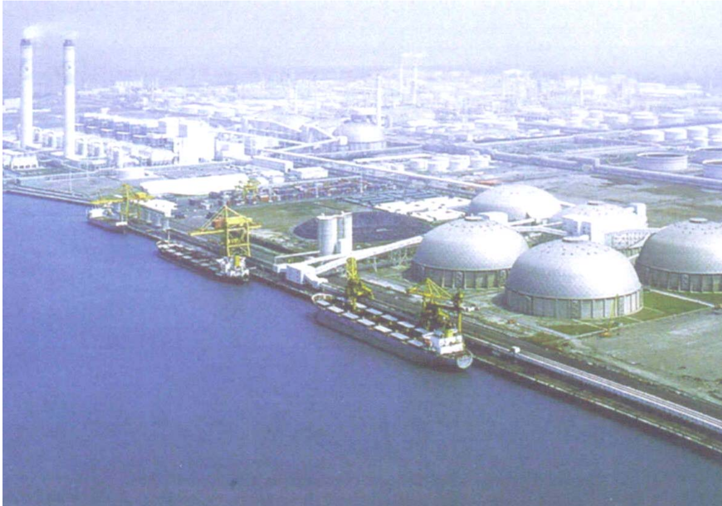
9 SCHADE Circular Storages at the FPC - Mai Liao Plant in Taiwan - 180,000 tons each
