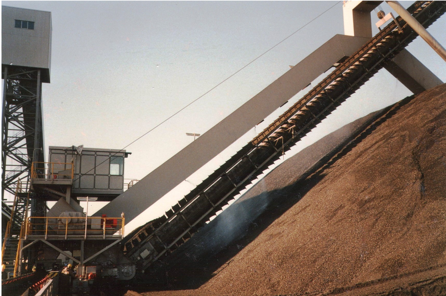
Portal Reclaimer (discharge via drag trough)
