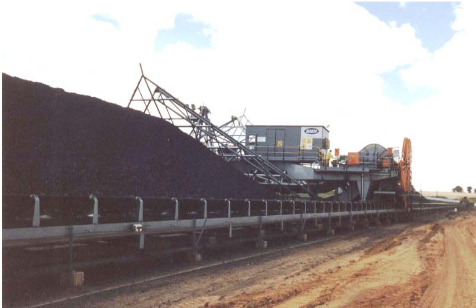
Bridge Reclaimer (discharge via drag trough)
