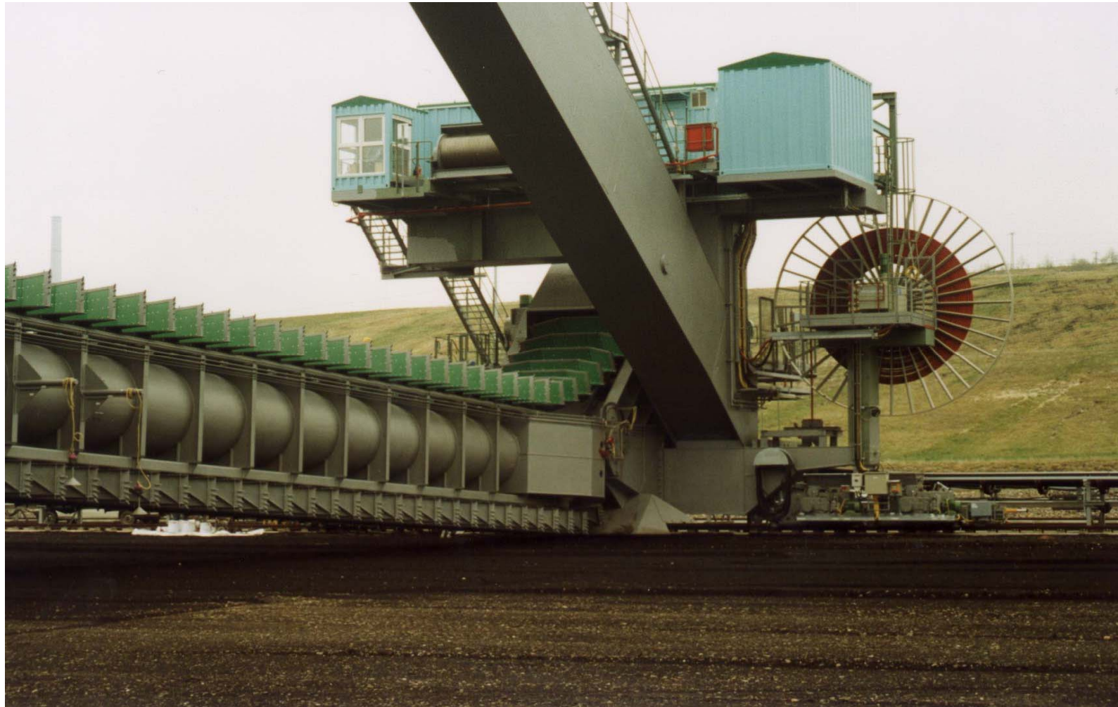
A-side view, showing boom, shovels, power supply
