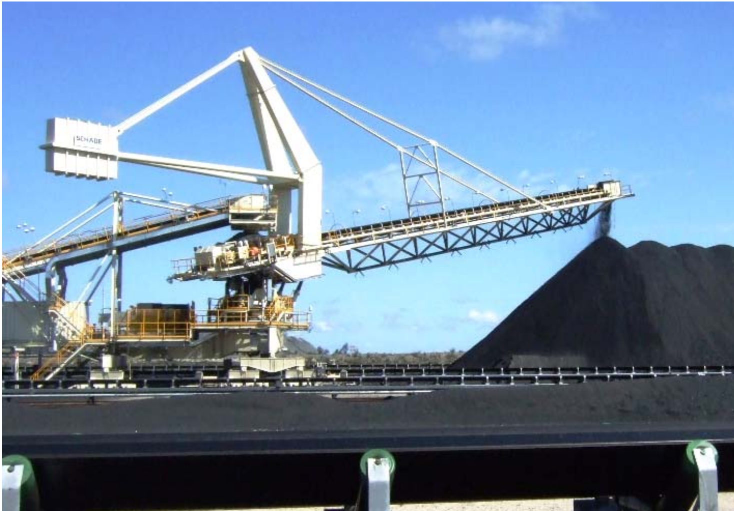
Stacker, slewing and luffing (hydraulic)
