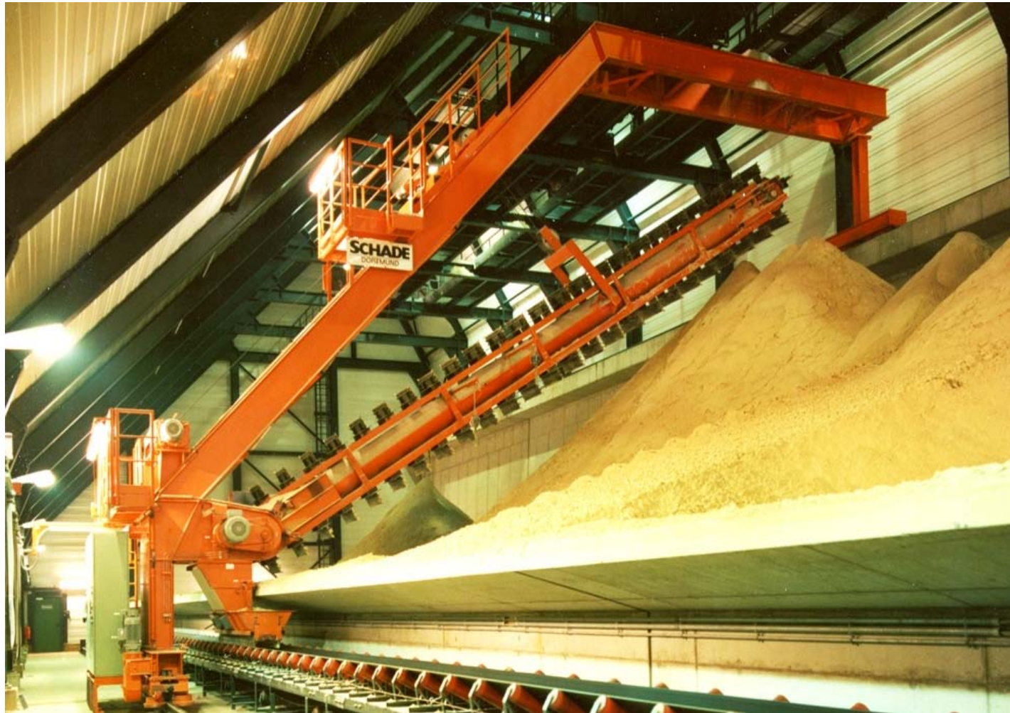
Semi-Portal Reclaimer (discharge via concrete ramp)
