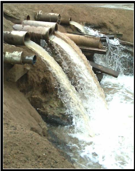
Bottom Ash Slurry Lines
