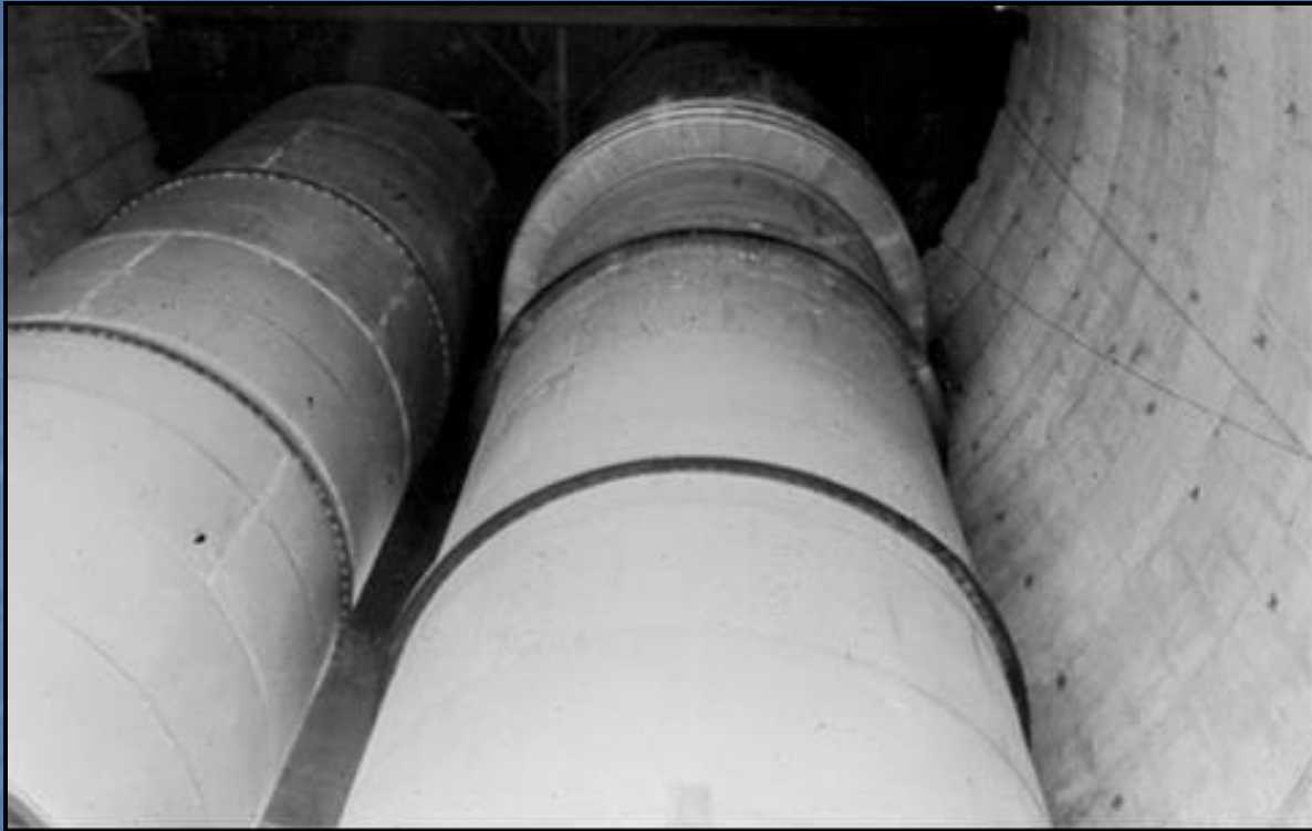
FGD chimney flues fabricated from solid NiCrMoNb alloy 625 plate
