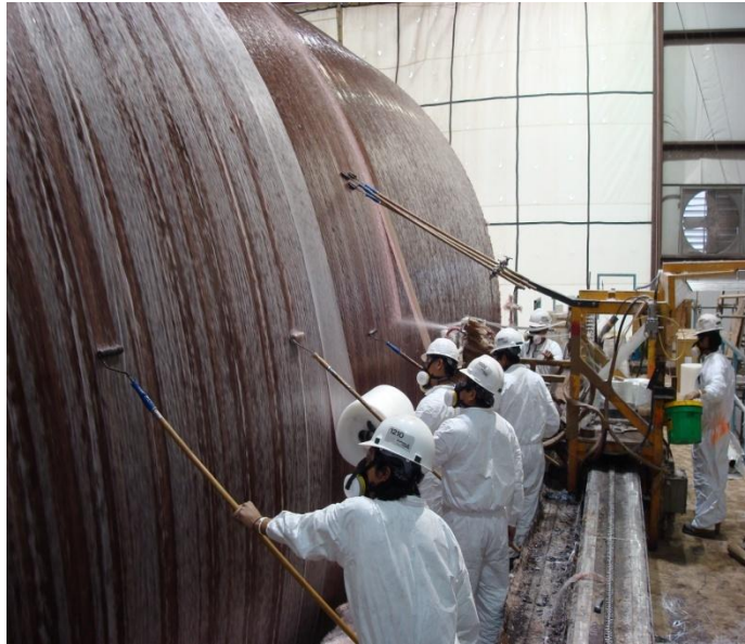
Fabrication shop on-site
