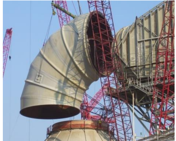
Working on field assembly
