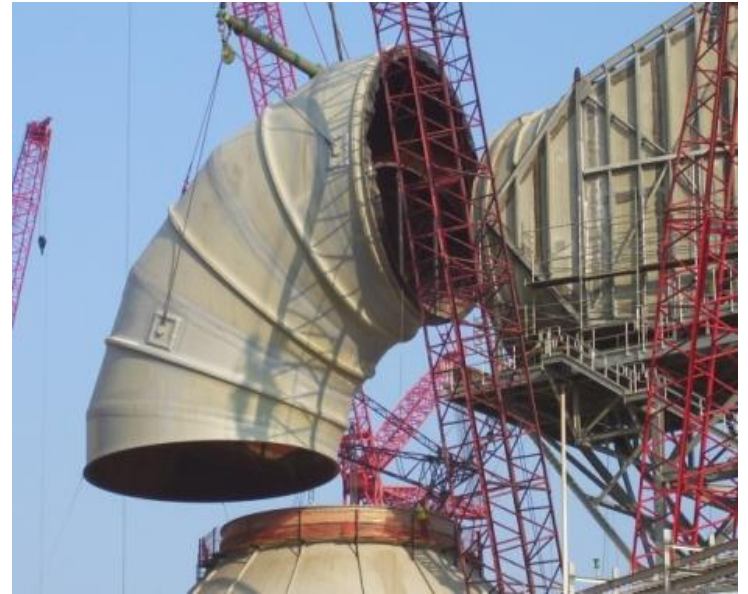
Working on field assembly
