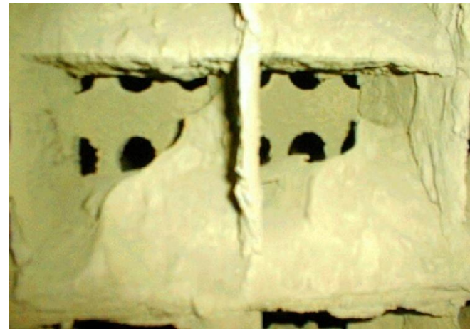
Source: Lehigh Energy Update June 2001. SCR AND SNCR PROCESSES INCREASE RISK OF AIR PREHEATER FOULING
