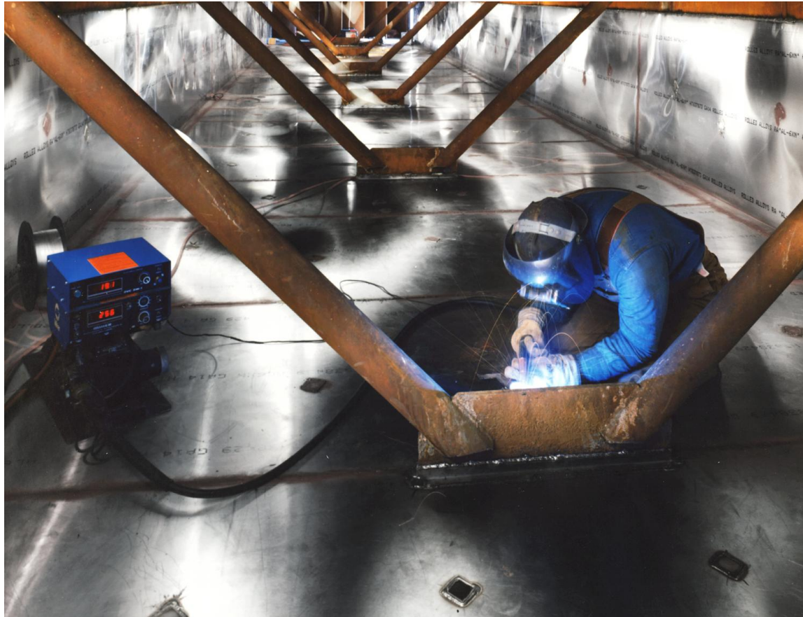
AL-6XN Bypass Duct Wallpapering at IP&L
