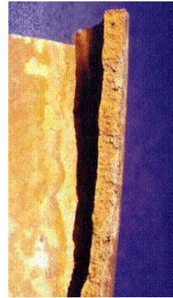
Through the wall tube failure and pitting due to bad chemistry
