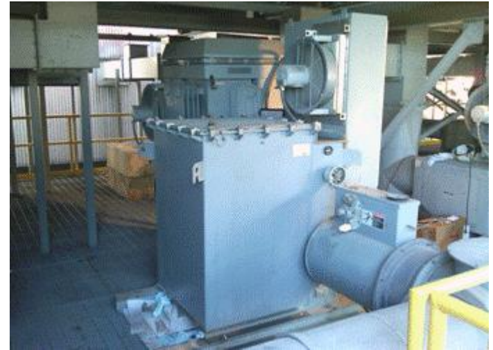
EPRIswitch HV SCR Stack Tank PowerPlus supply in background Plant Barry Inlet Field
