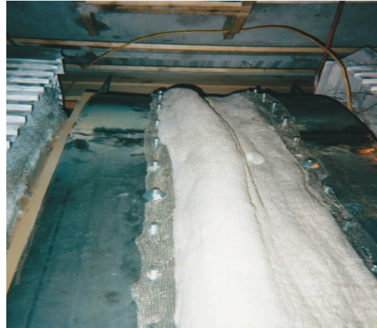
B) Protective layer installed.
