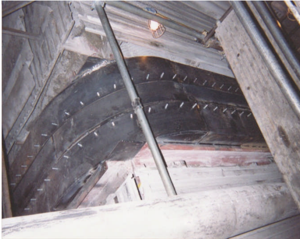
A) Metal frame [studded] welded in place
