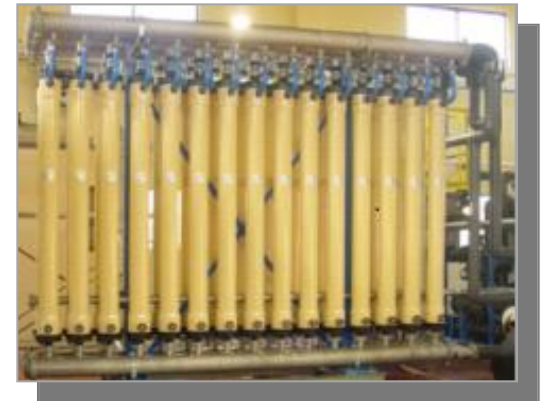
Pall system in slipstream of recirculation ( 5%; 80 m 3 /h)
