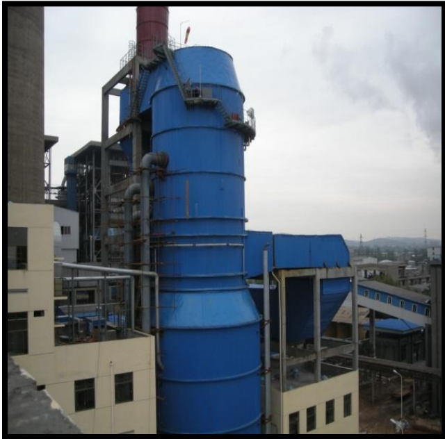
Qilu Thermal Plants Shandong Province, China
