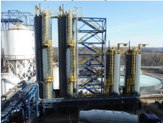
DSI and ACI Mercury Scrubber System
