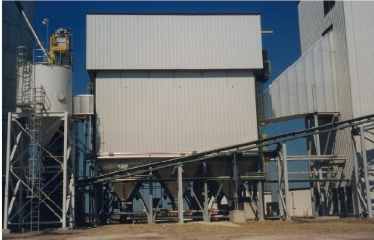
Coal Fired Boiler Baghouse 220,000 ACFM @ 420 F
