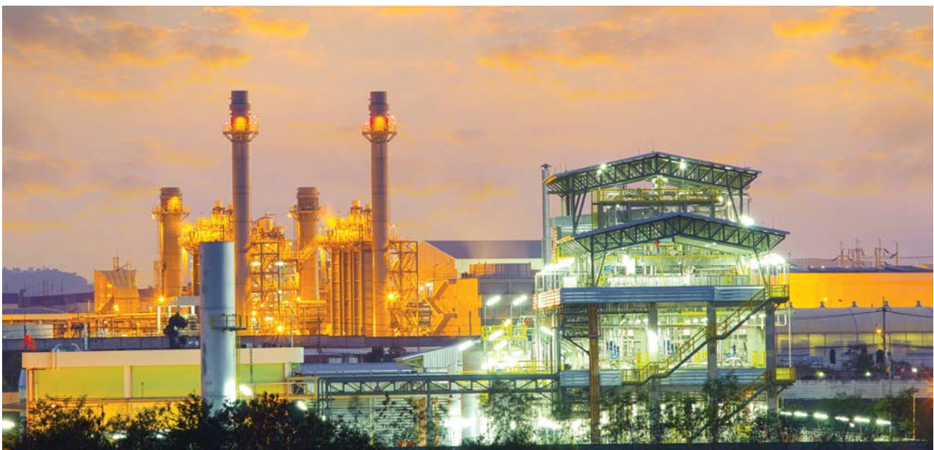
Natural gas combined-cycle power plants require much less water to produce a megawatt of electricity than coal or nuclear plants. Image courtesy of Pulsafeeder.
