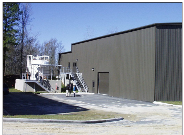
Filter operation includes addition of methanol to filter influent to provide organic substrate for a denitrifying microbiological culture in the filter media. Methanol is stored in an 8000-gal. tank.
