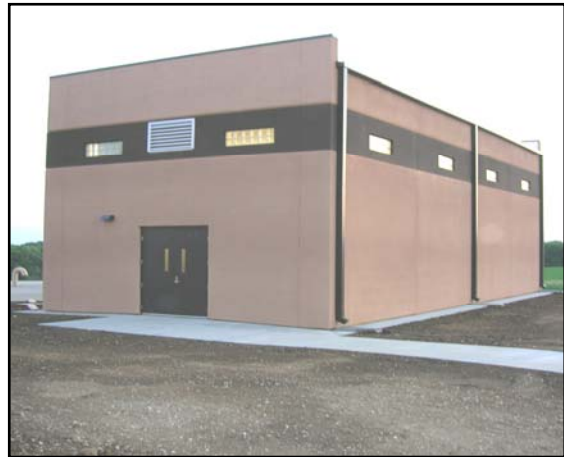
The water treatment plant in Papillion.
