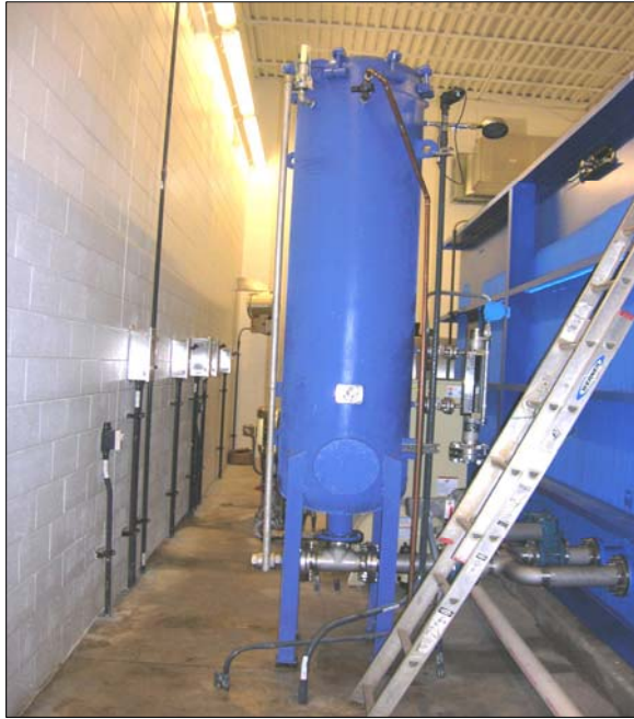
The Clari-DAF system saturator.
