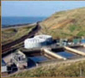
WHITEHAVEN WWTW, UK In collaboration with Galliford Northern, ITT constructed a Sanitaire Intermittent Cycle Extended Aeration System (ICEAS) for North West Water's first four basins ICEAS Sequencing
