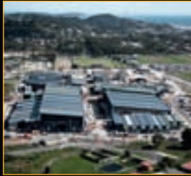
GOLD COAST, QUEENSLAND, AUSTRALIA ITT was contracted to supply a Leopold Desalination Pretreatment System to Queensland Australia. As part of the Gold Coast Desalination Project, the first large
