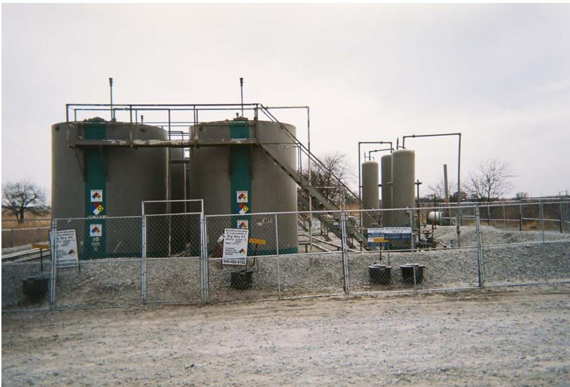
**Figure 2-1. Example Storage Tank Battery with Separators**
