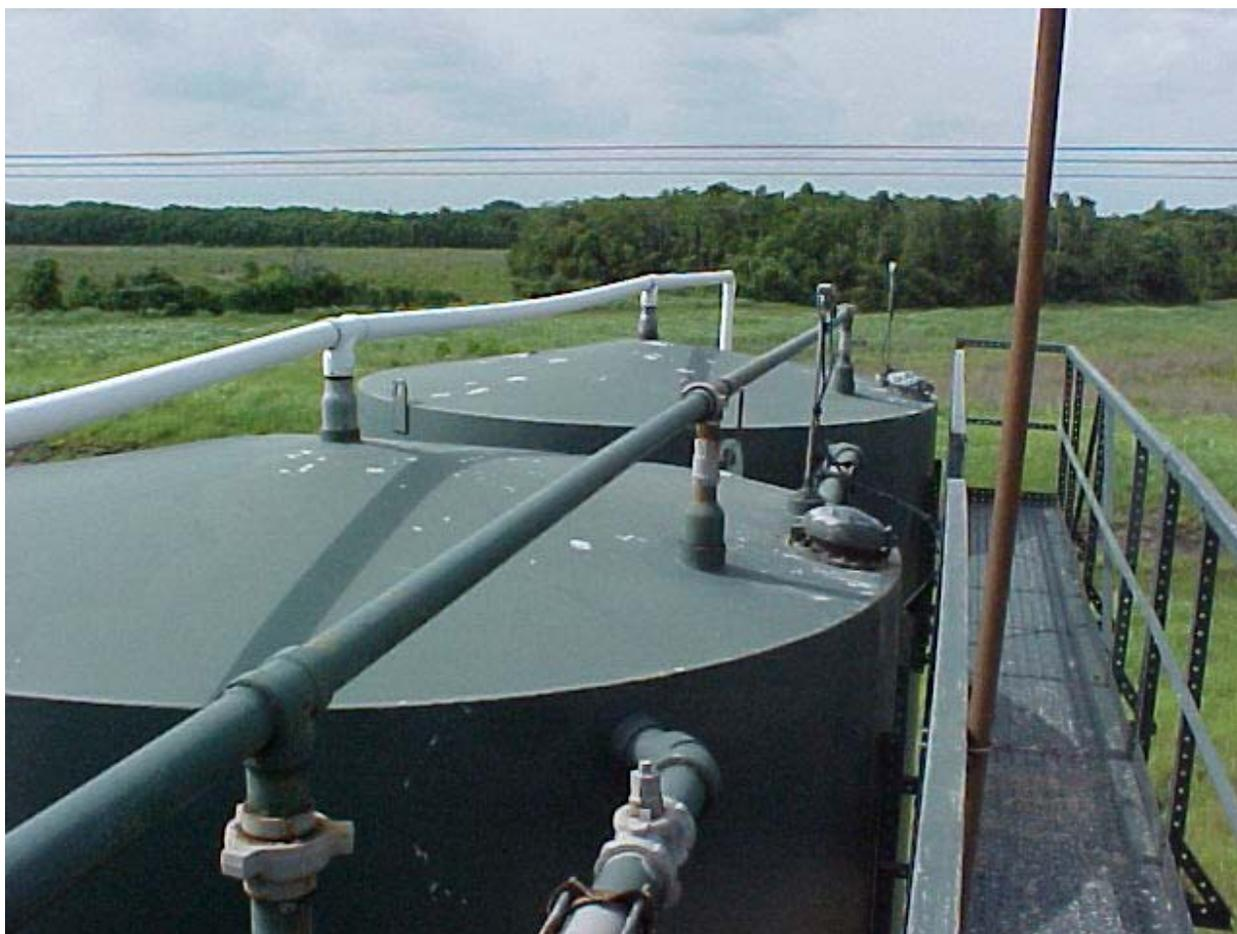
**Figure 2-2. Vent Gas Gathering Pipe atop Storage Tanks**
