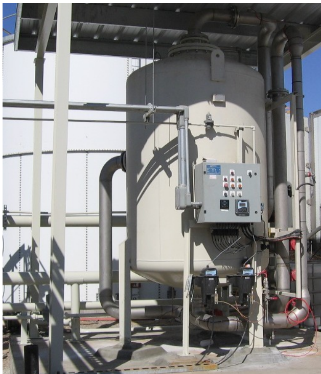
Figure 3 - Current Single Micro Media Filter
