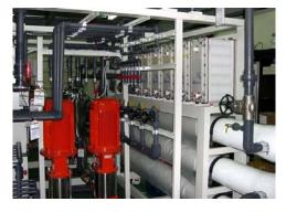
1-pass RO can be enhanced using GTM (e.g., Liqui-Cel<sup>®</sup>) for even better EDI performance. GTM can reduce the  $CO_2$  which enhances EDI performance, reduces scaling potential, and helps SiO<sub>2</sub> removal by the EDI.
