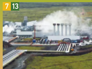
Geothermal Power Plant
