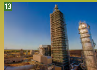
CO 2 Recovery Plant
