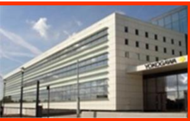
Yokogawa Europe (The Netherlands)
