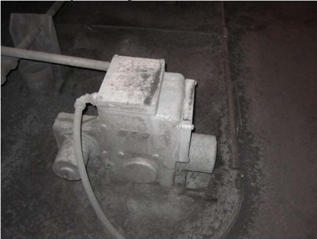
Electric controller (prone to freezing)
