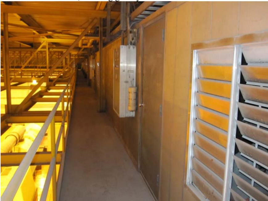
Front of A-Line Fans, showing gravity louvers
