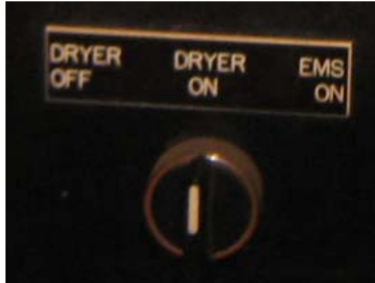
Figure 7: Operating desiccant dryer set to "Dryer On" mode. Set to "EMS On" after ECM implementation
