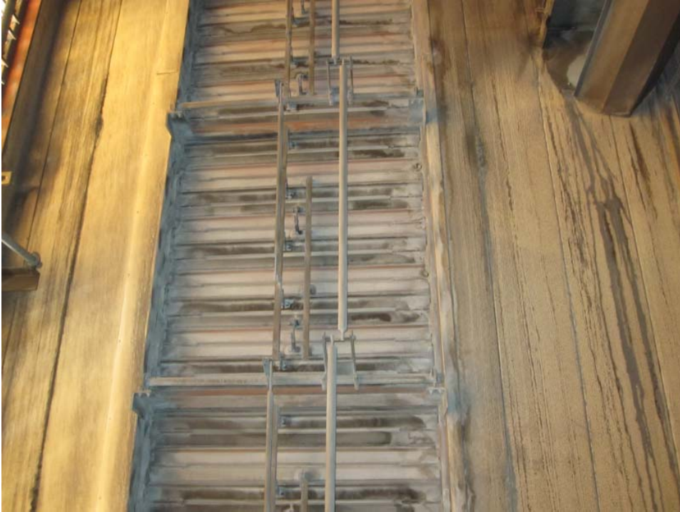
Intake Louvers for warm, recycled air
