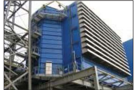
Figure 1: AAF Power & Industrial's H12 HEPA final stage filters behind canisters (left)
