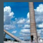
Removal of the kiln stacks at the Darra plant Photo: CAPL
