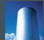
Cement kiln exhaust stack Photo: CAPL
