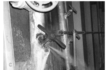
The hazardous effects of high pressure wire draw and the breakdown of torque seated sealing can create safety concerns and jeopardize the effectiveness of power generation.
