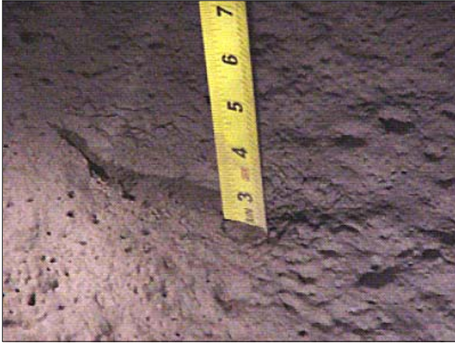
Figure 5 Horizontal flue inspection.
