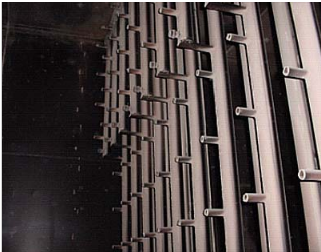
Figure 6 Somerset AIG inspection December 2001.
