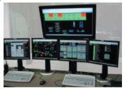
"Originally," he continued, "Units 1 and 2 were housed in one control room, while Units 3, 4 and 5 were housed in a separate control room. As part of this project, we combined these into one. The new system has worked so well, that we now utilize one control operator to run both Units 1 and 2, where before each unit had a dedicated control operator assigned to each unit."
