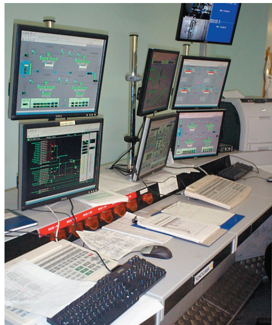
CENTUM CS 3000 station operator consoles
