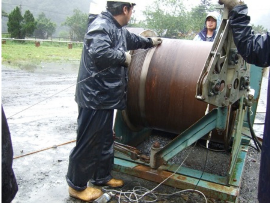
Above – Winding and spooling of stainless steel fiber optic cable
