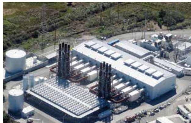
Humboldt, Eureka, California (10 x Wärtsilä 18V50DF, 162 MW) The multi-fuel DF engines can operate on light fuel oil as back-up. The plant is equipped with combined SCRs and oxidation catalysts and meets the strict Californian emission requirements both in gas and liquid fuel mode.
