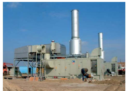
Air intake system being installed at a new compressor station
