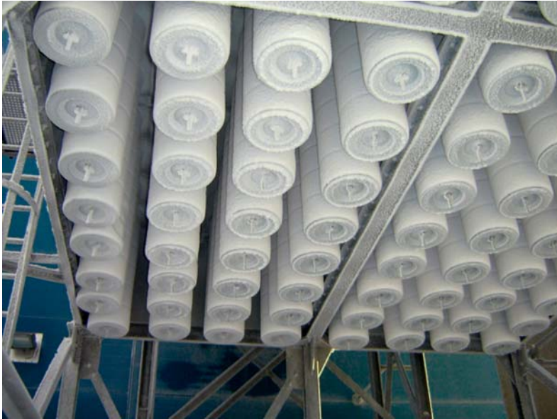
TFP 95 depth-loading filter cartridges function reliably at temperatures of down to -35^{\circ}\text{C} thanks to porous ice layers
