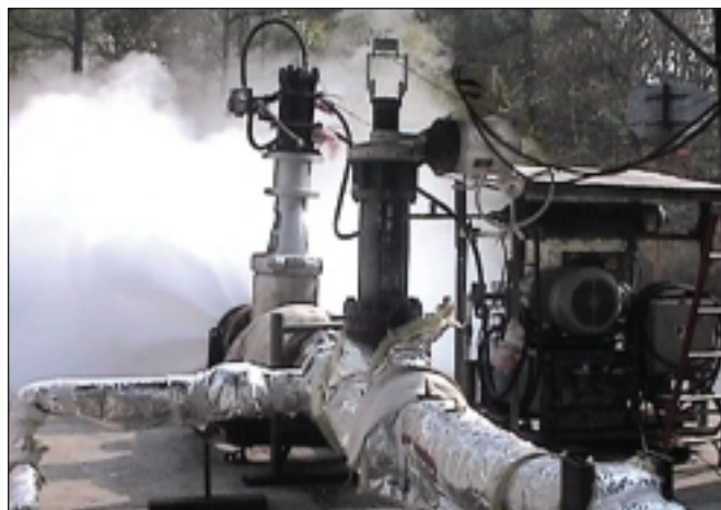
Loop isolation and blowdown test with hot pressurized water of Velan electrically actuated 8" Class 900 regular port loop isolation valve. The water flashes to steam in a starburst pattern as it blows down to atmosphere.
