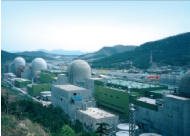
Yonggwang nuclear power station in South Korea. Velan valves are installed in many of South Korea's nuclear power stations.
