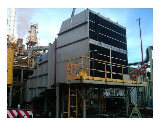
Installation of Clark Air Systems project using Munters DH2100 Mist Eliminators with filter bank and vessel to extend the life of the filters and reduce pressure loss. PCS Nitrogen Trinidad
