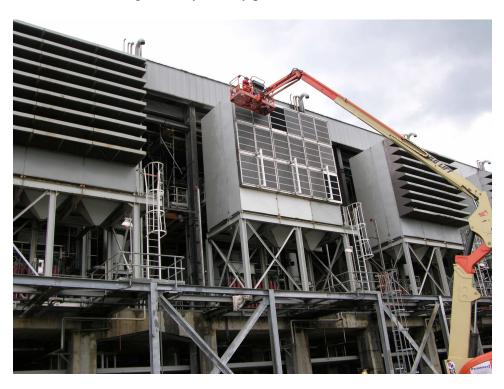
Installation of Munters DH2100 Mist Eliminators with Framework to extend the life of the filters and reduce pressure loss. Atlantic LNG Trinidad
