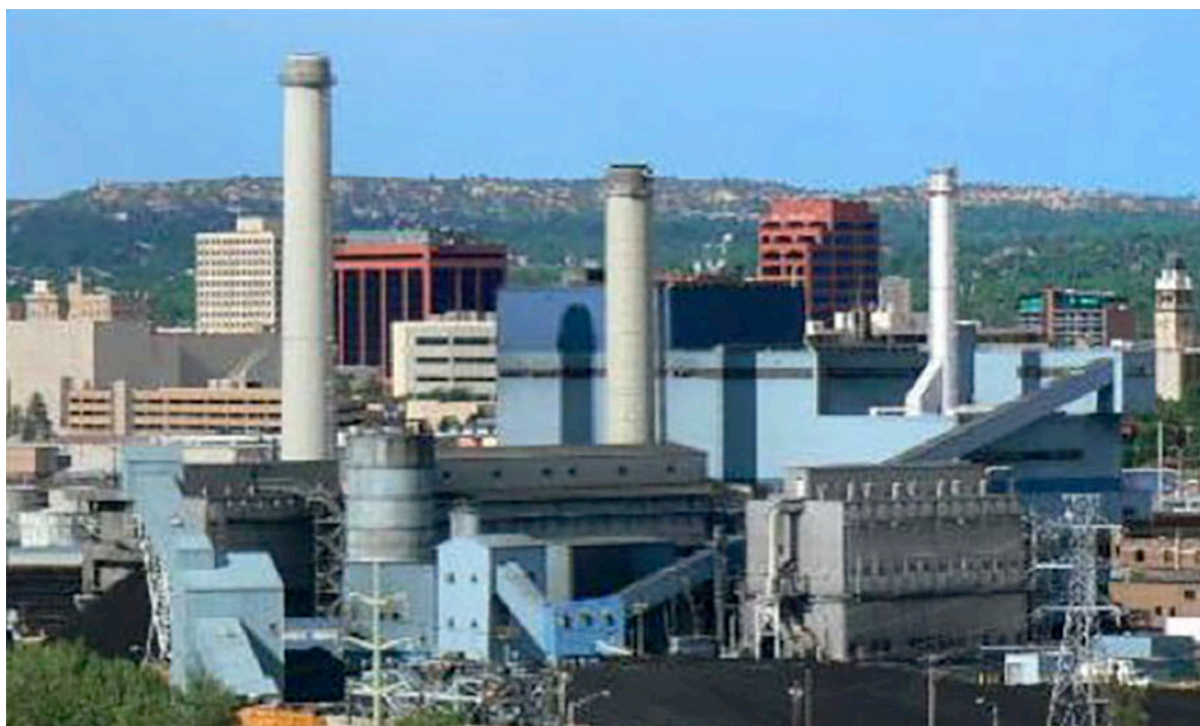
Figure 7 $110 million NeuStream™ plant at the Martin Drake Power Plant, CO, USA (Neumann, 2014)
