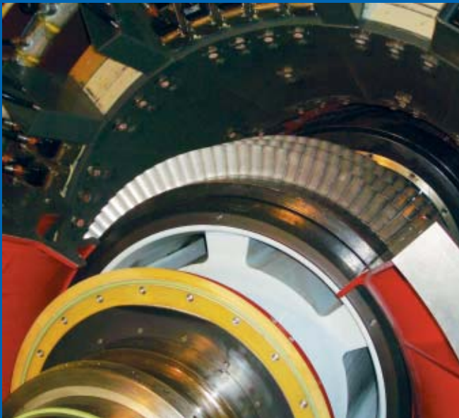
Generator stator and rotor as well as the generator fan and H2 tubes during reassembly.
