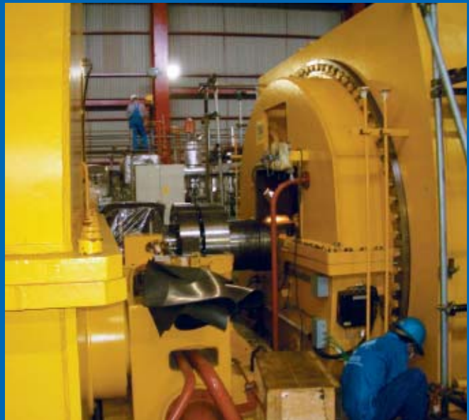
Turbine rotor and generator rotor ready mating together after alignment checks.
