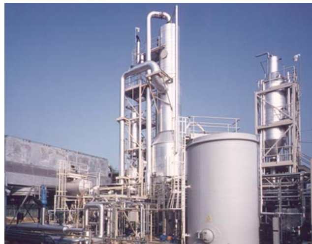
Figure 5: Typical Steam Driven SAGD ZLD System
